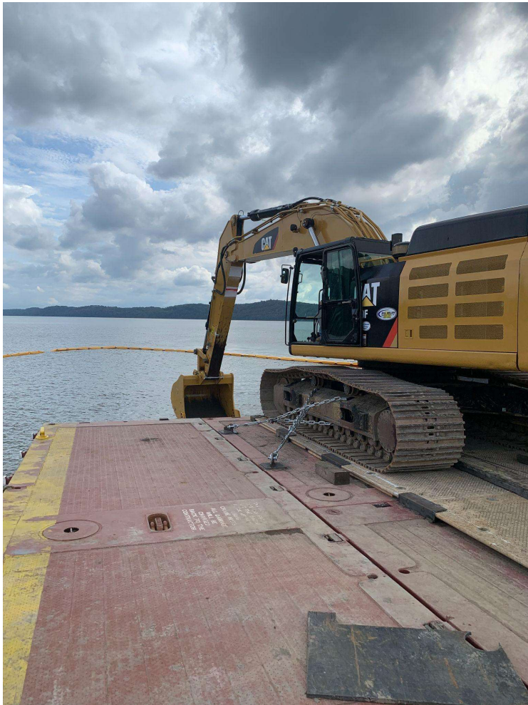
Figure 12: Dredging component of Maryland Innovative Reuse and Beneficial Reuse Pilot.
