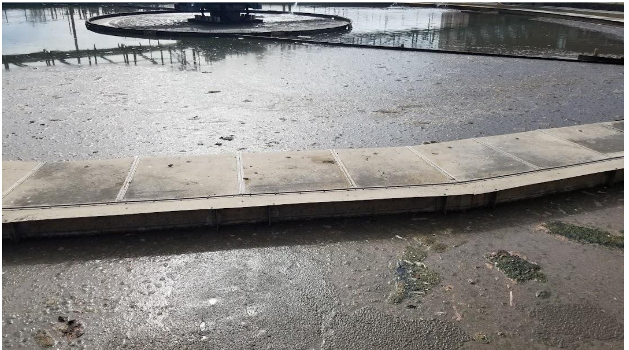
Figure 5c: Scum on the water surface at both sides of the launder cover within Clarifier # 5a.
