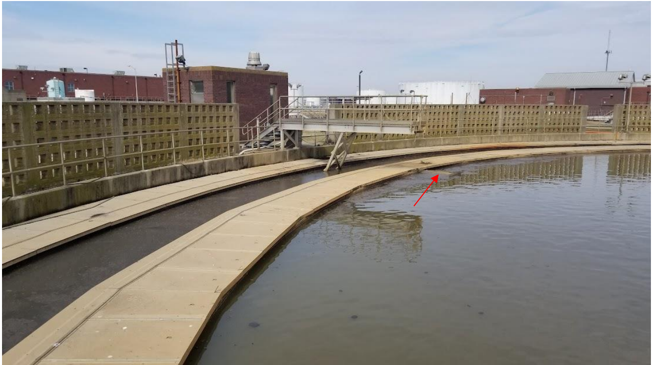
Figure 5b: Surface of the scum trough (pointed with a red arrow) at the same level as the water surface within Clarifier #4.
