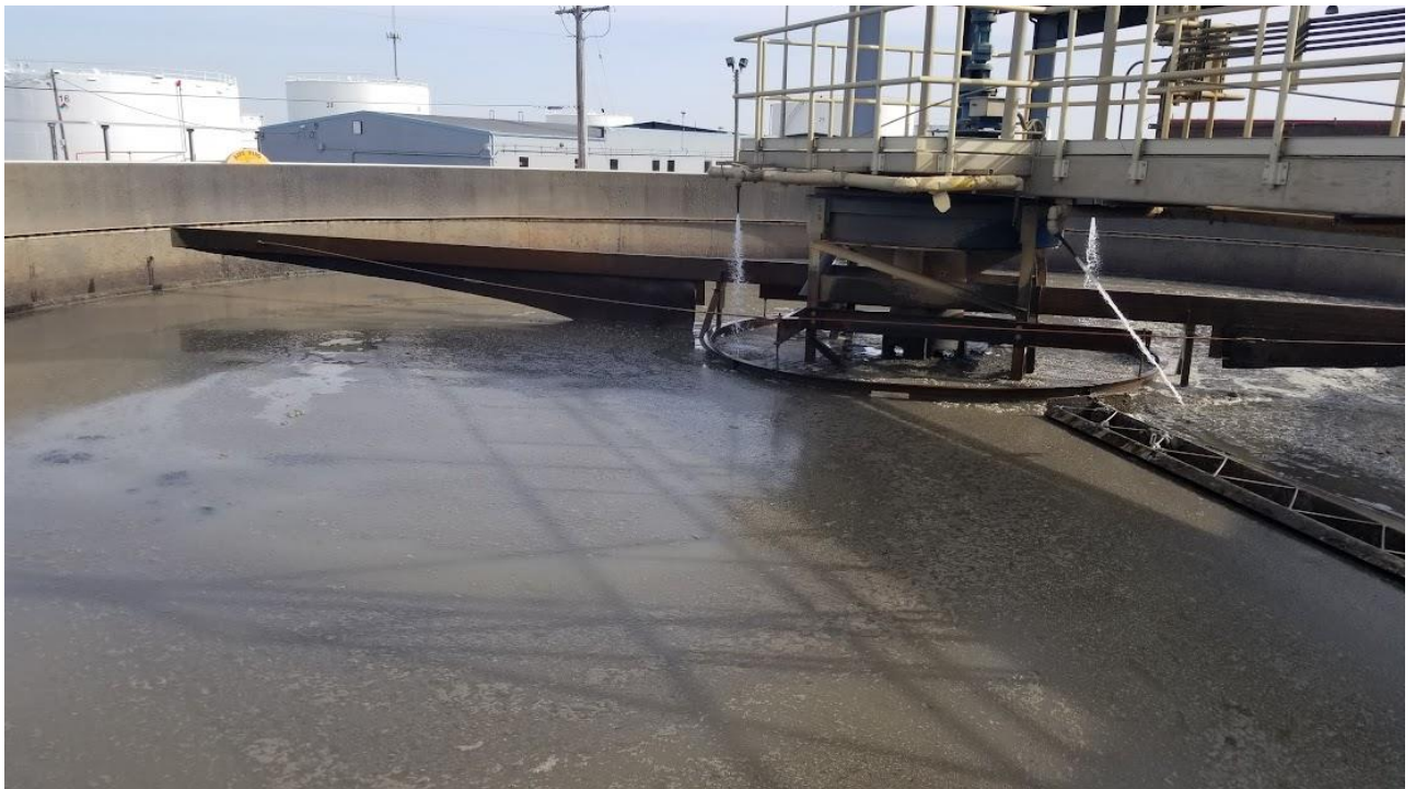
Figure 2d: Scrapper arm above the water surface within GST #2.
