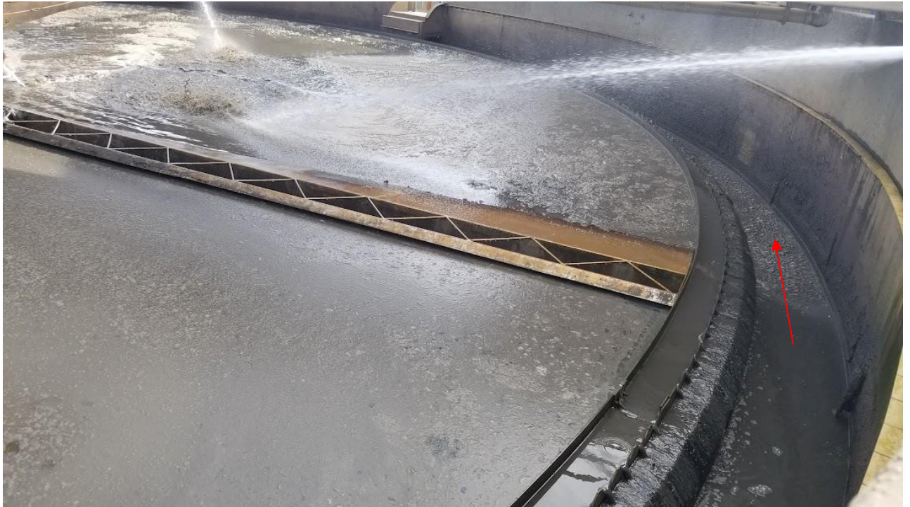
Figure 2a: Sludge at the surface of GST #1 and next to the outer side of the weir (pointed with a red arrow).
