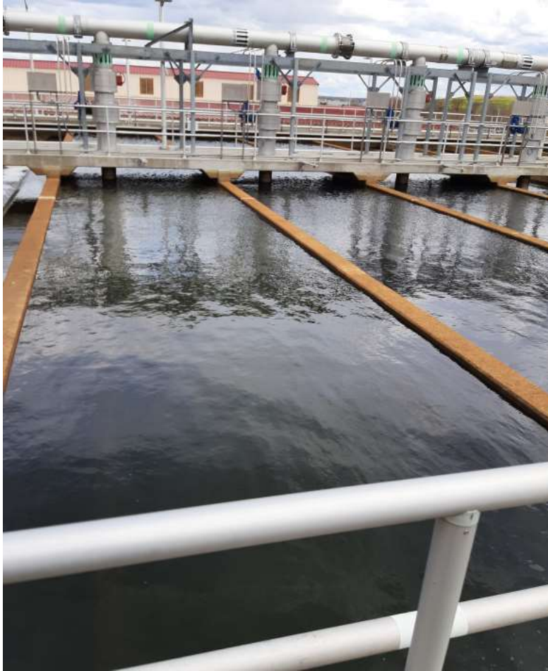
Submerged DN filters 3/26/22
