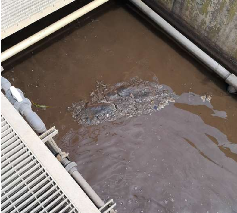
Floating solids in one of the reactors 3/26/22
