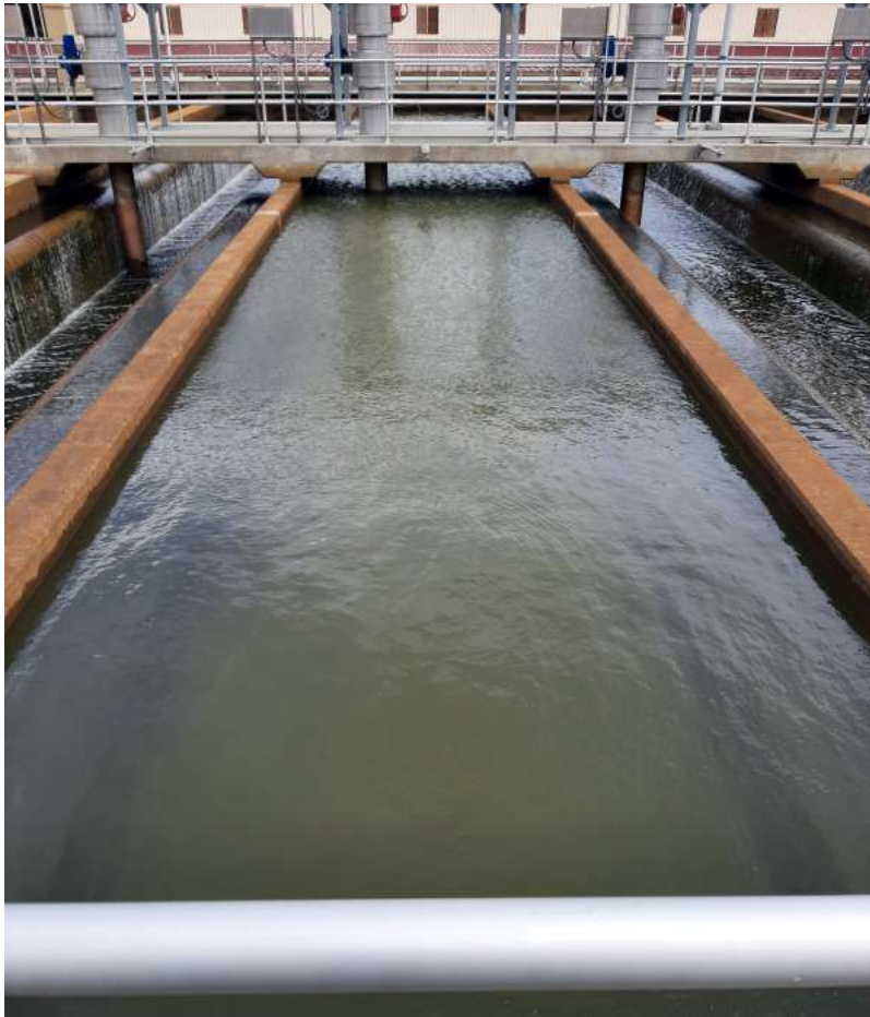
3/26/22 submerged DN filter
