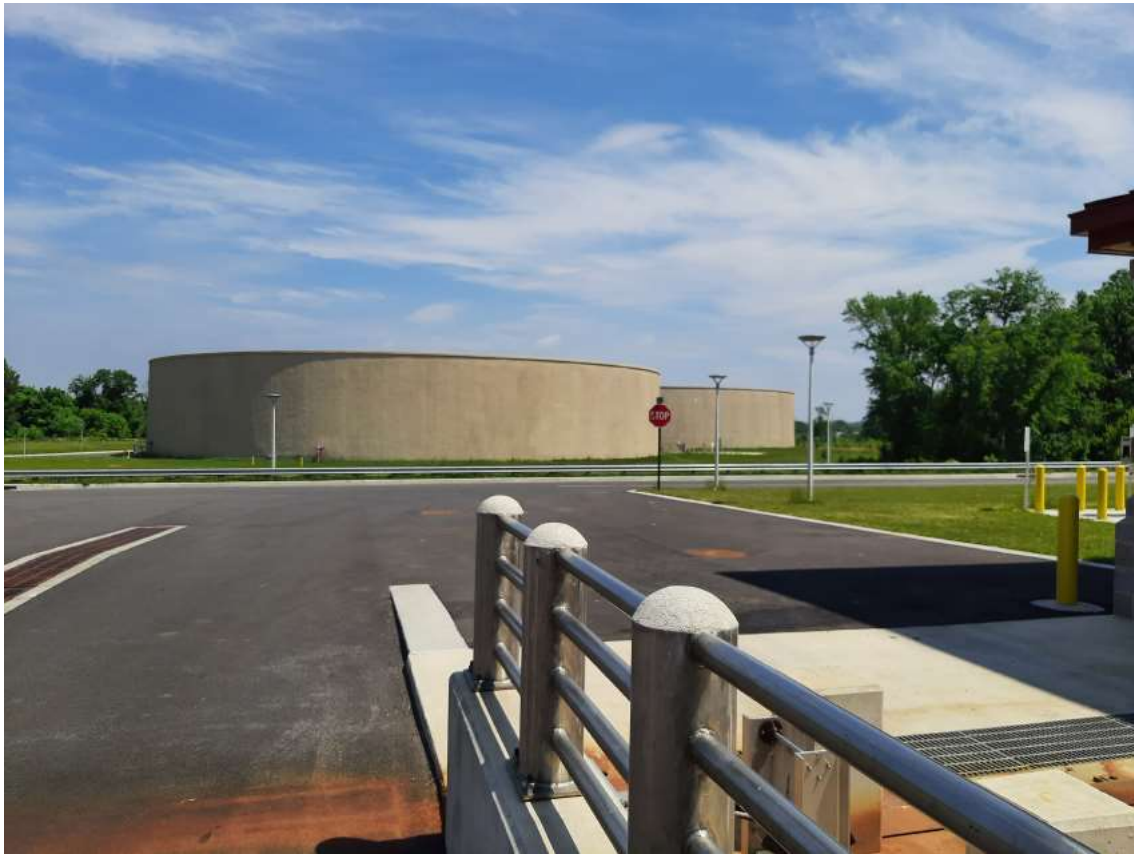
6/2/22 Flow equalization tanks
