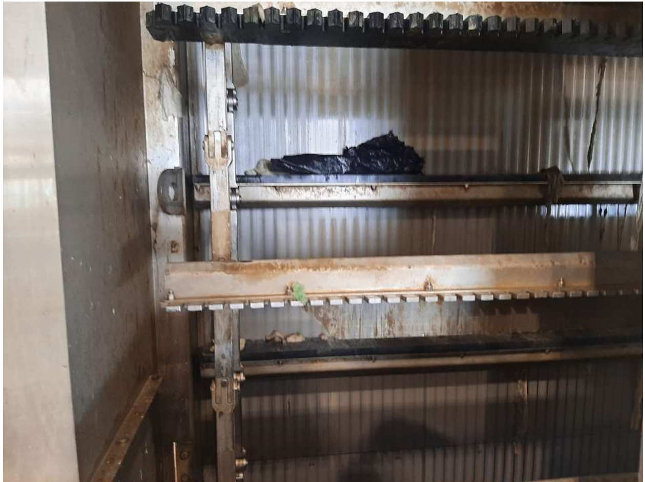
1/26/23 Active coarse screening unit
