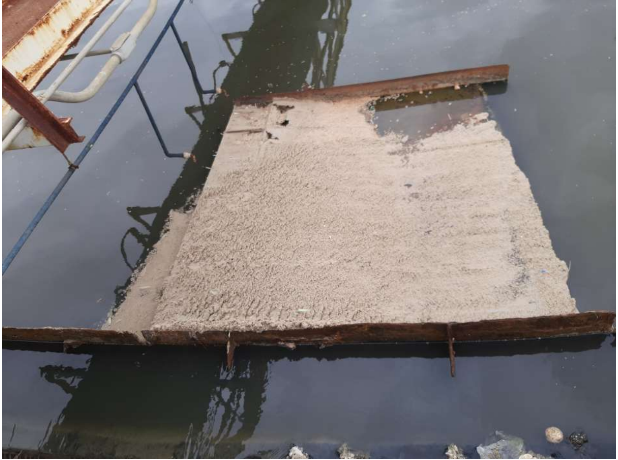
1/26/23 PST#1 scum trough clogged with FOG and scum. The scum trough should be cleaned out and scum pit pumped out as necessary.
