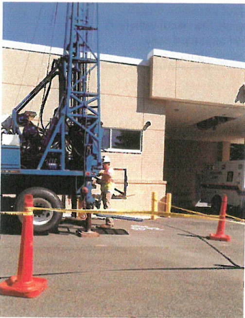
MW-52 is located south of the Emergency Room Ambulance Entrance.
