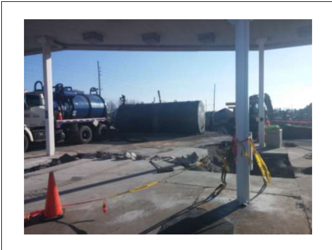
Photograph 6: Piping and disperser removal
