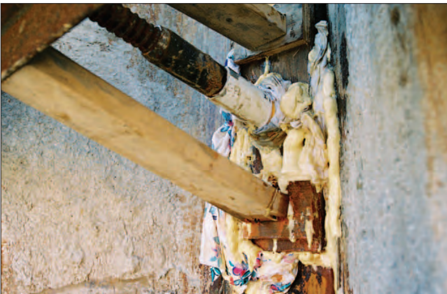
Tieback sealed with HYDRO ACTIVE® CUT
