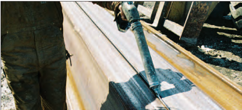
Swellseal® WA applied with caulking gun
