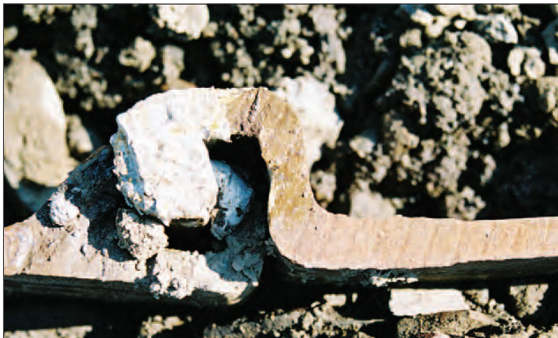
Swellseal® WA after driving sheet piles
