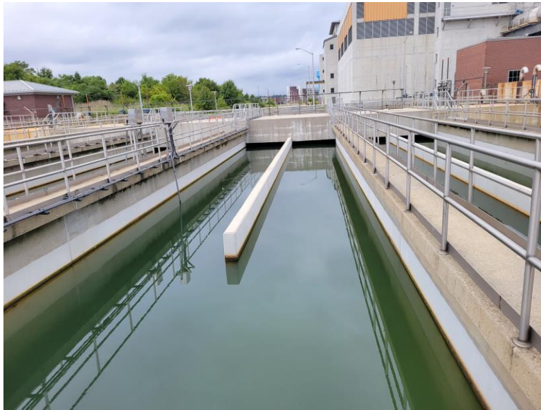
Image 10: Final pass of Contact Chamber #1.
