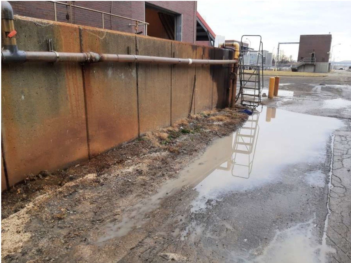
1/30/23 spilled lime and water mixture.
