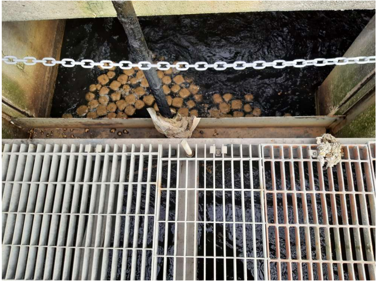
1/30/23 Floating slugs of FOG in the channel leading to the biological reactors.
