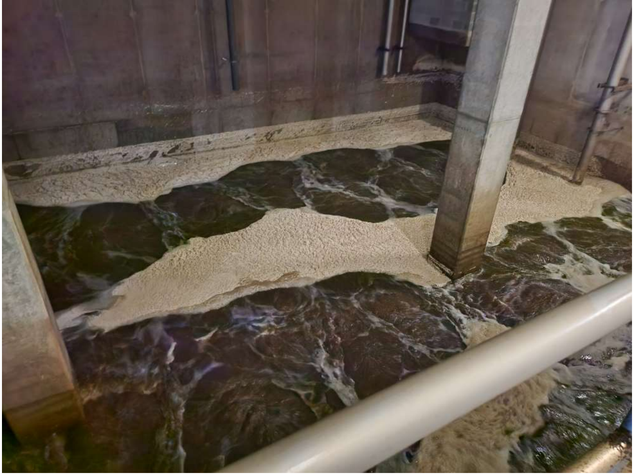
1/30/23 Picture taken today of backwash mud well showing media accumulation. See picture below showing mud well condition on 11/2/22.
