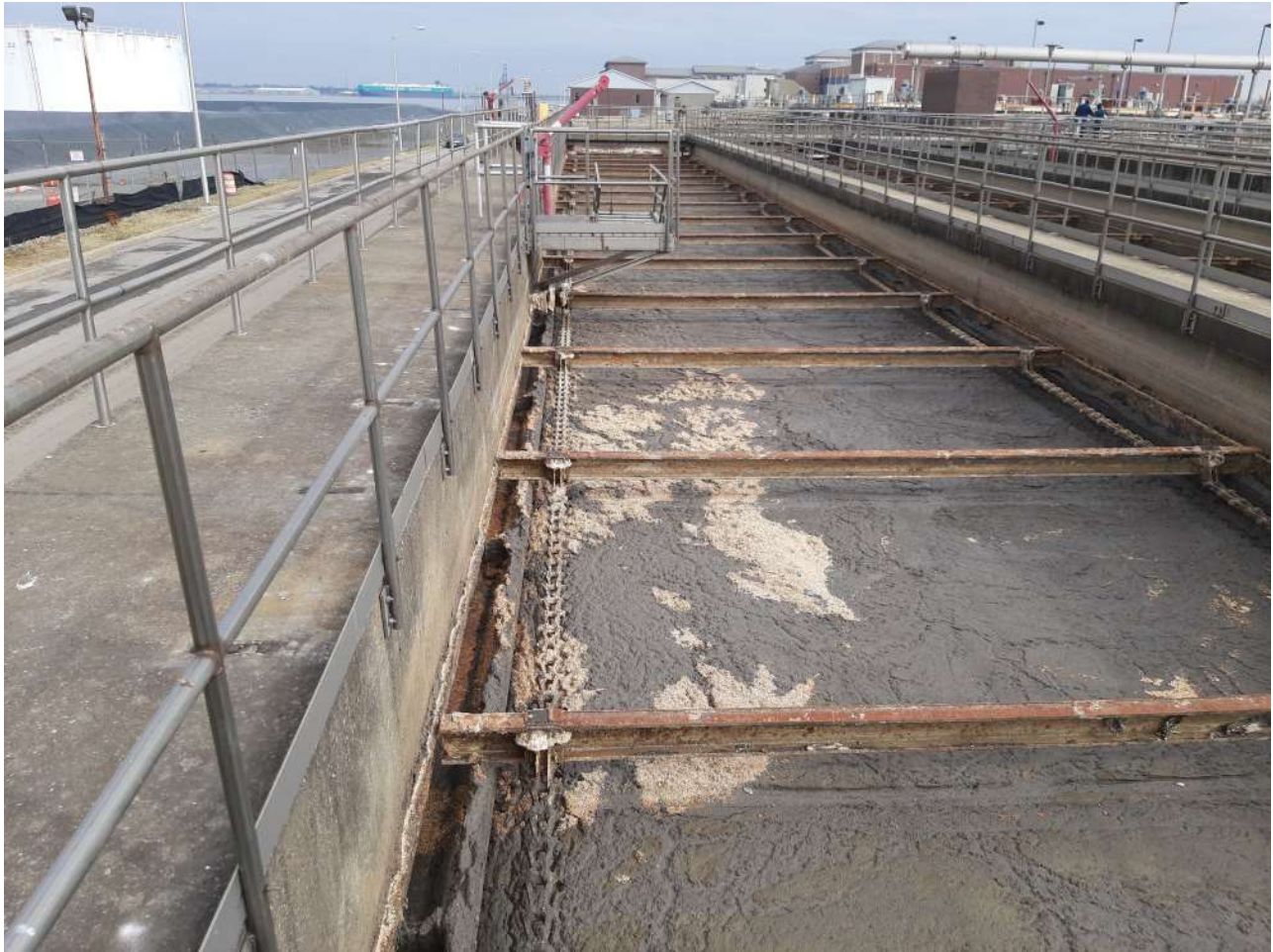
1/30/23 Thick layer of FOG on the PSTs
