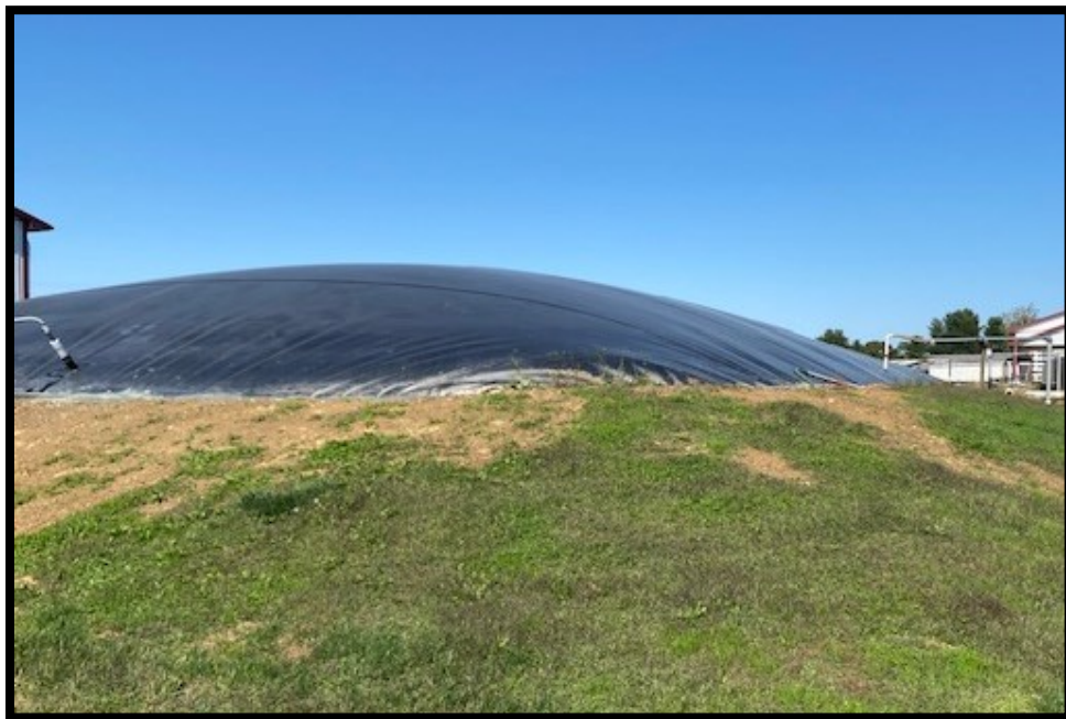
Anaerobic digester at Kilby Farm, Colora, MD
