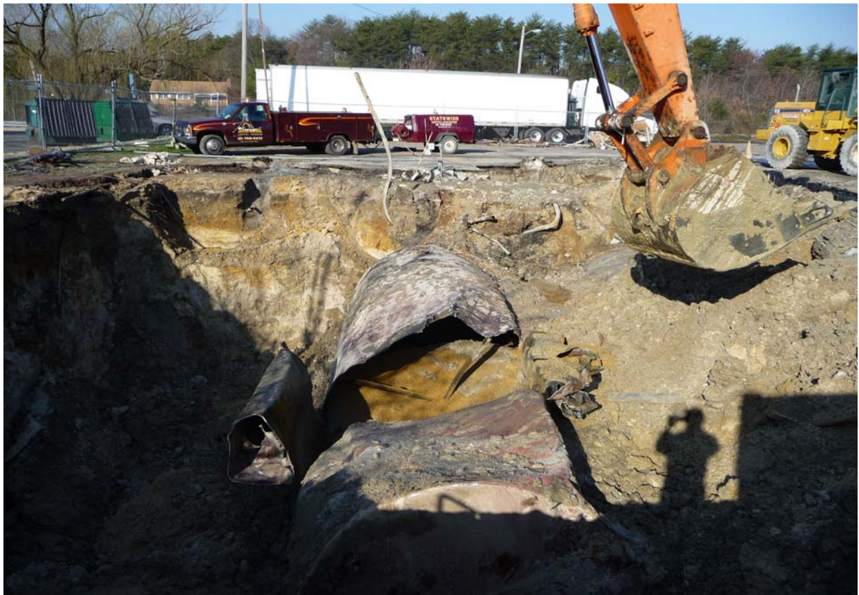
Photo of Tank 3 showing pea gravel contained in the tank.
