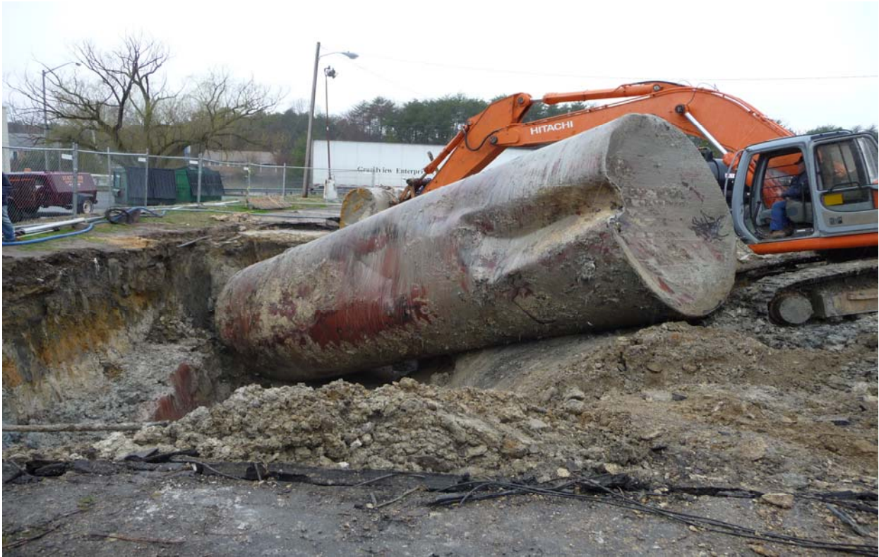
Photo of Tank 1 being removed from the excavation.
