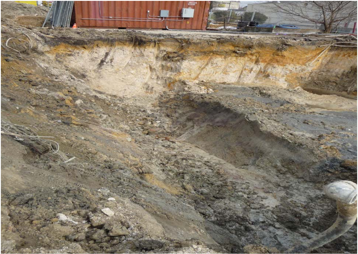
Photo of excavation cavity after removal of Tank 2.
