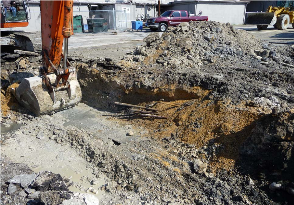
Photo showing the top of Tank 4.
