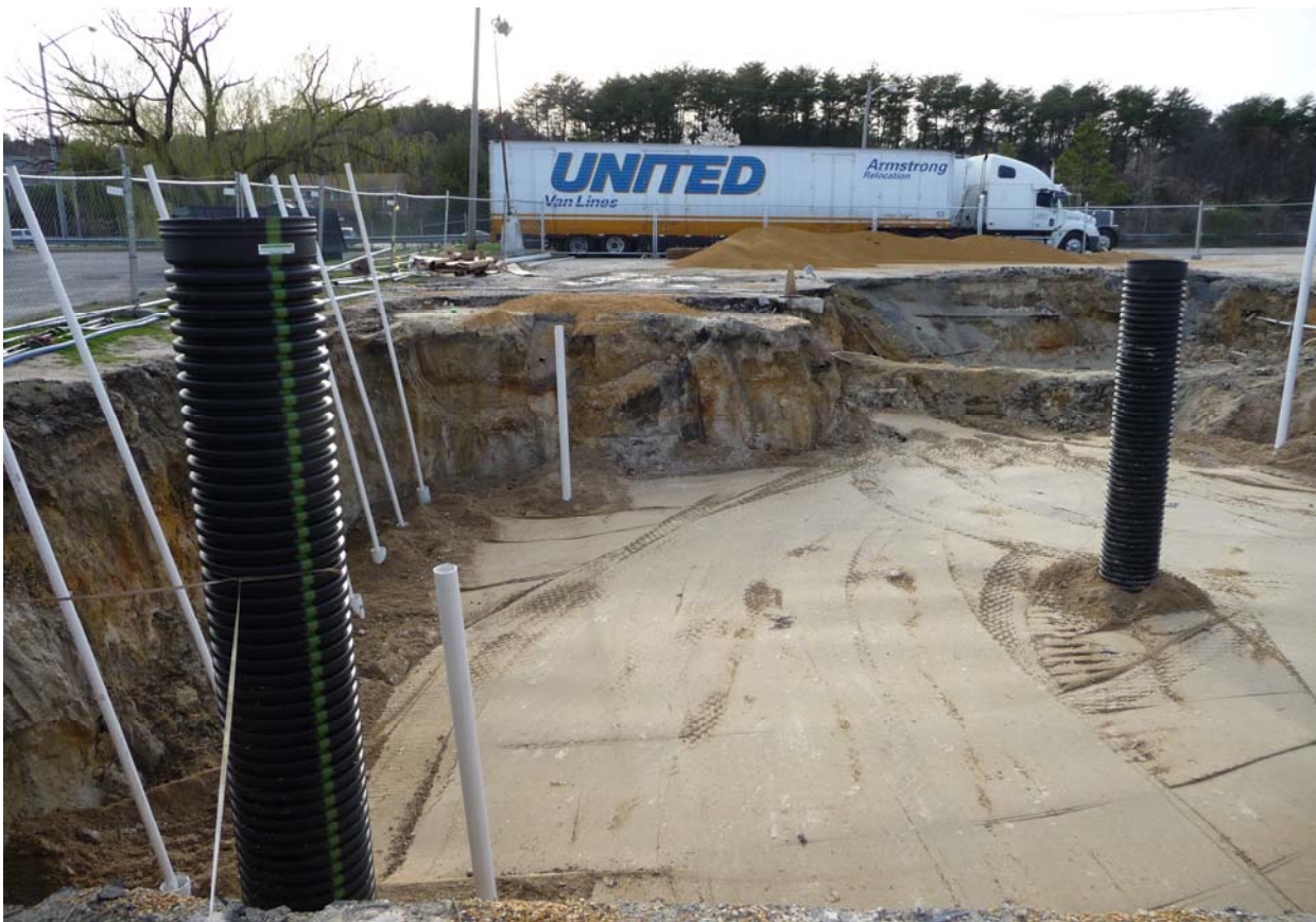
Photo showing backfill being installed in tankfield excavation.
