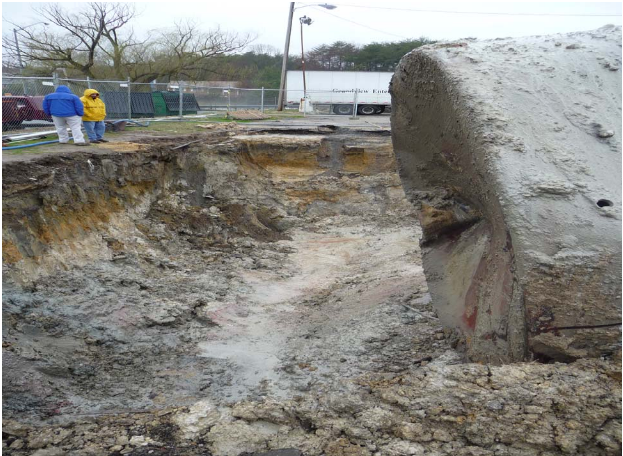
Photo of excavation after removing Tank1.
