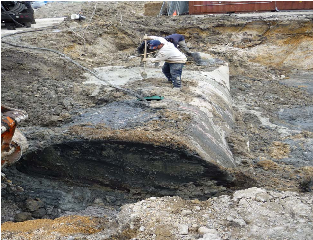
Photo of Tank 2 partially exposed and being pumped of remaining fluids.
