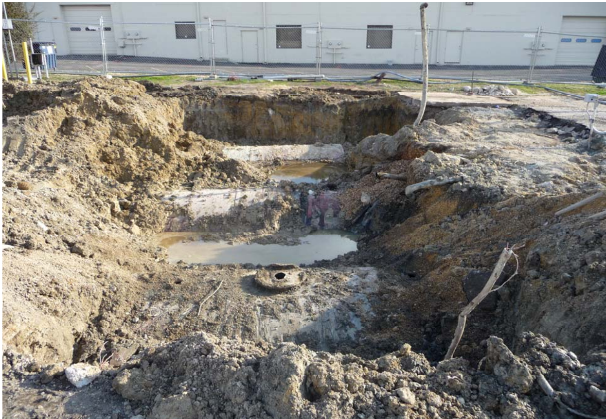
From foreground – Tanks 2, 3 and 1 partially exposed
