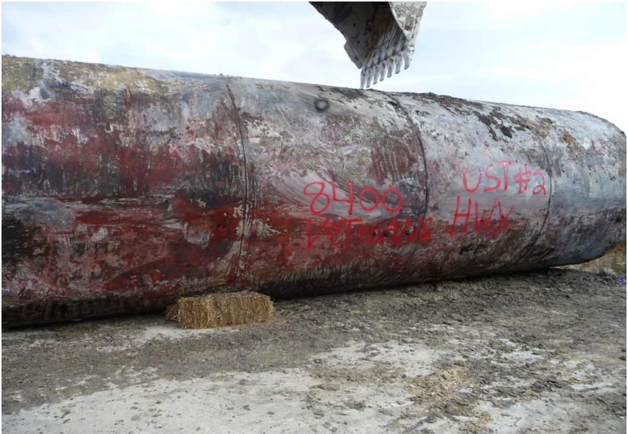
Photo of Tank 2 being prepared for transport from the site.
