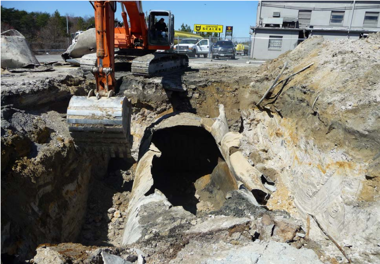
Photo of Tank 4 with top removed and pea gravel contents exposed.
