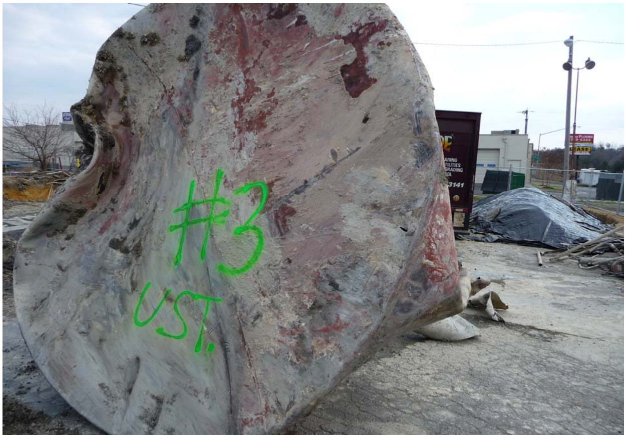
Remnant of Tank 3 after being remove from the excavation.
