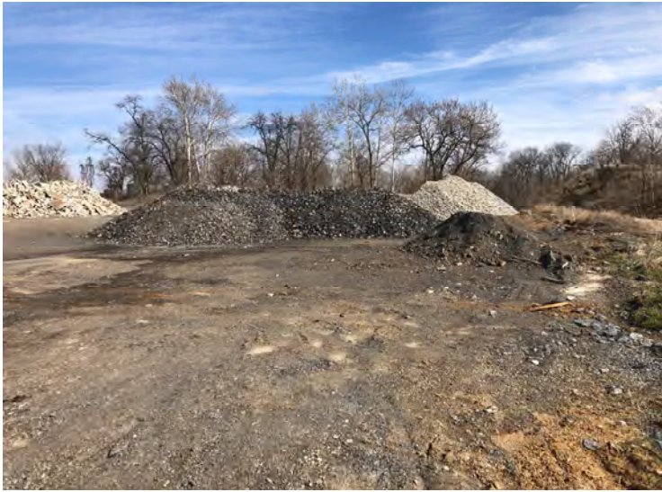
Photo 13: View of stockpiles of concrete, asphalt, stone, and cement located on the western portion of the Site. East of East Street.
