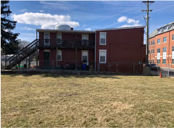
Photo 17: View of western portion of the Site. West of East Street.
