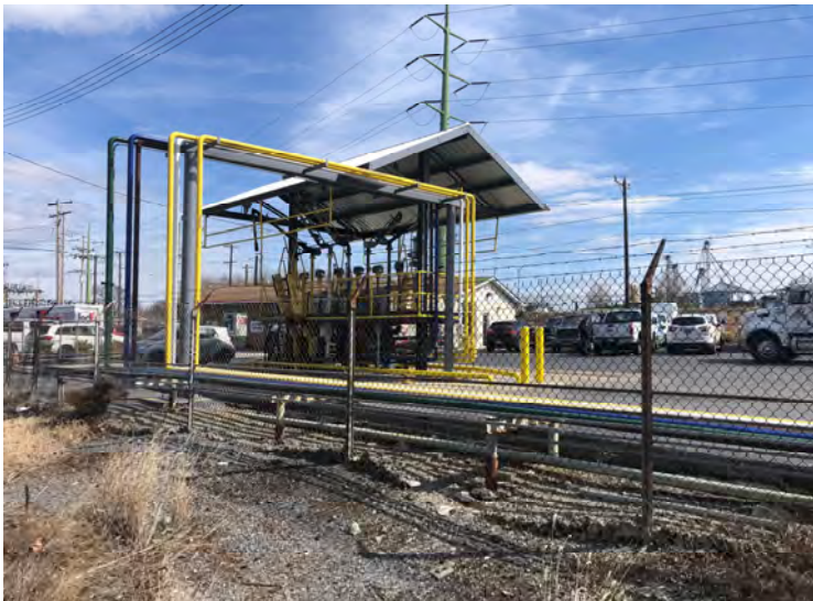
Photo 27: View of adjacent property to the northeast.
