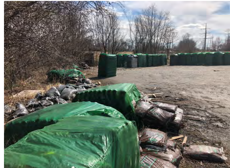
Photo 4: View of pallets of mulch located in the northern portion of the Site.
