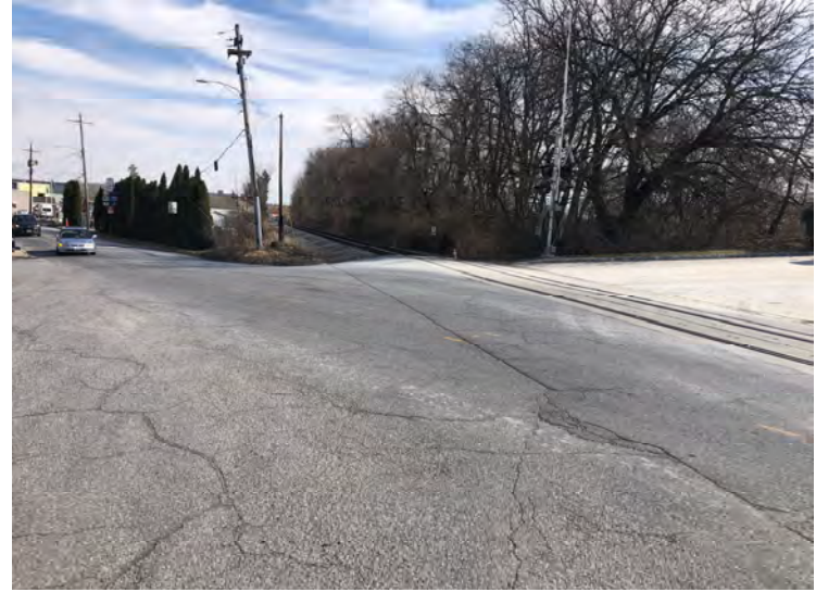
Photo 26: View of railroad tracks extending onto the eastern portion of the Site.
