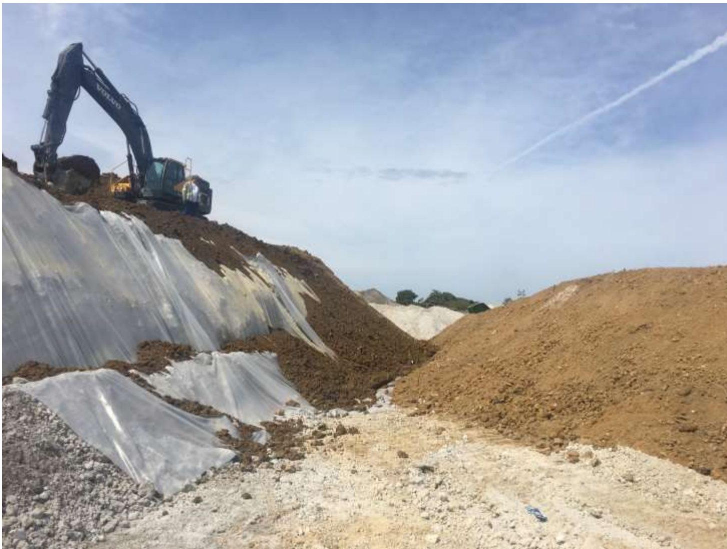
Capping slag excavation face and contaminated slag pile with plastic and clean fill
