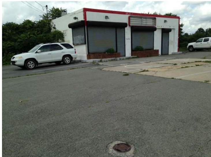
Photo 14: Overview of 5600 Ager Road (former Ager Road Citgo). Note the former dispenser island to the right. The UST field was located to the left of the building.
