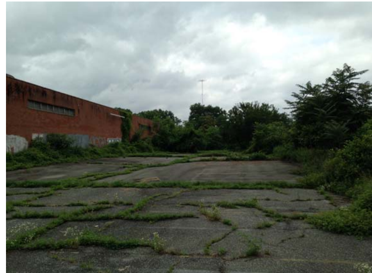
Photo 4: View of eastern façade and parking area of vacant warehouse.
