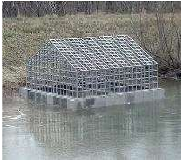
Welded Galvanized Steel Trash Rack (Top Mount)
