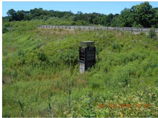
Metal Control Structure with Wooden Inserts
