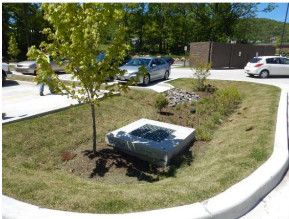
Control Structure in a Bioretention Filter
