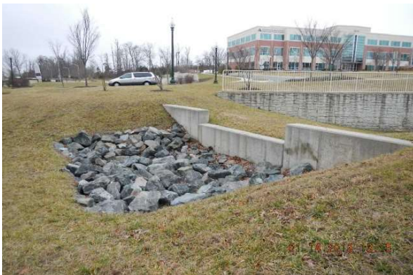
Concrete Weir (Photo courtesy of SWM, LLC)
