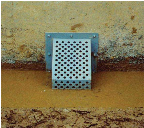
Low-Flow Orifice Trash Rack
