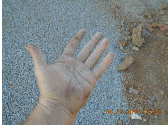
Residue/Dust from Unwashed Aggregate
