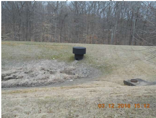
Metal Control Structure with Trash Rack
