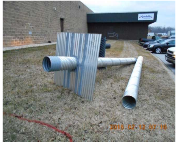
ALCCMP Pipe and Anti-Seep Collar
