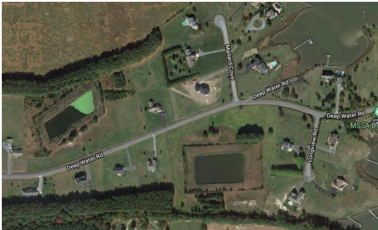
Aerial view of Deep Water 1 and 2 BIPs (left and bottom) near Little Choptank River (upper and lower right). Note proximity to tidal wetland transitions and surface water.
