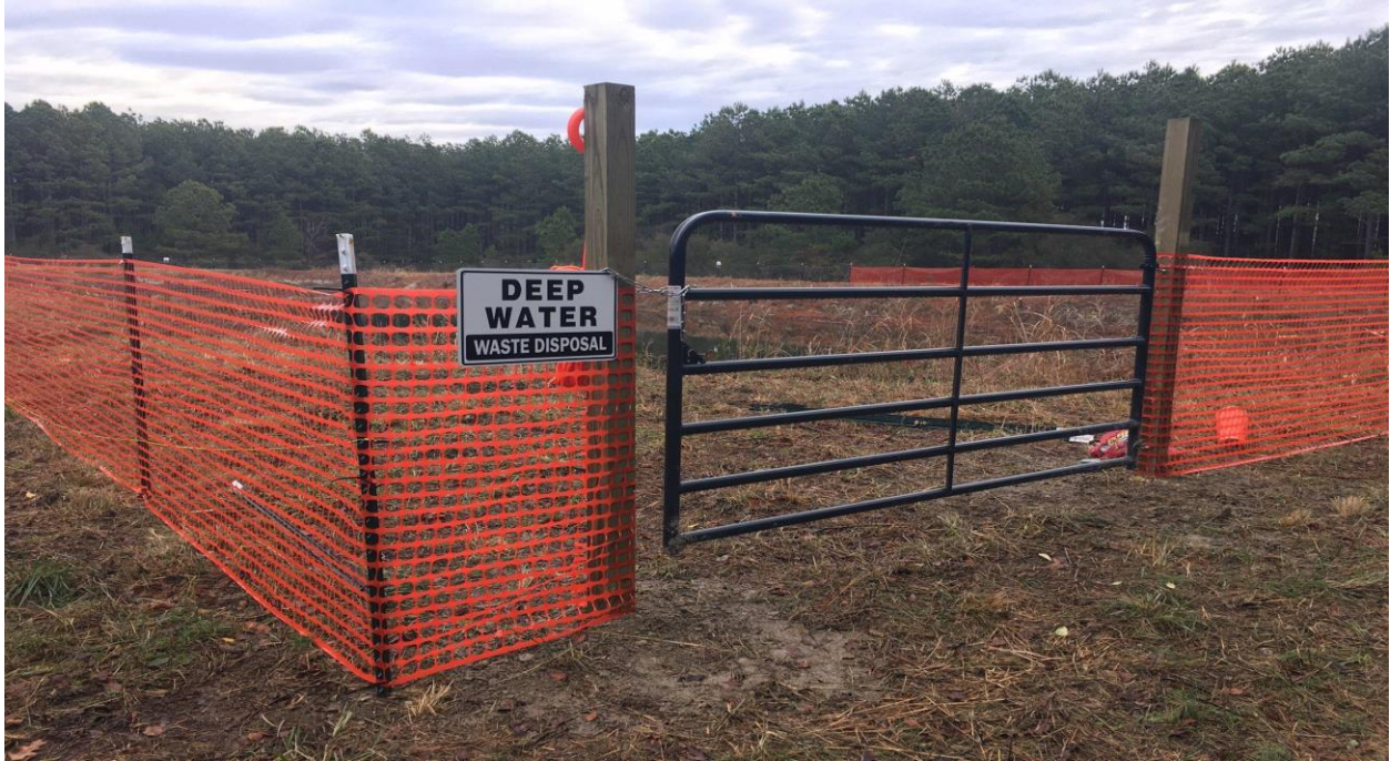
BIP with temporary fencing and adequate gate, signage, and life ring.
