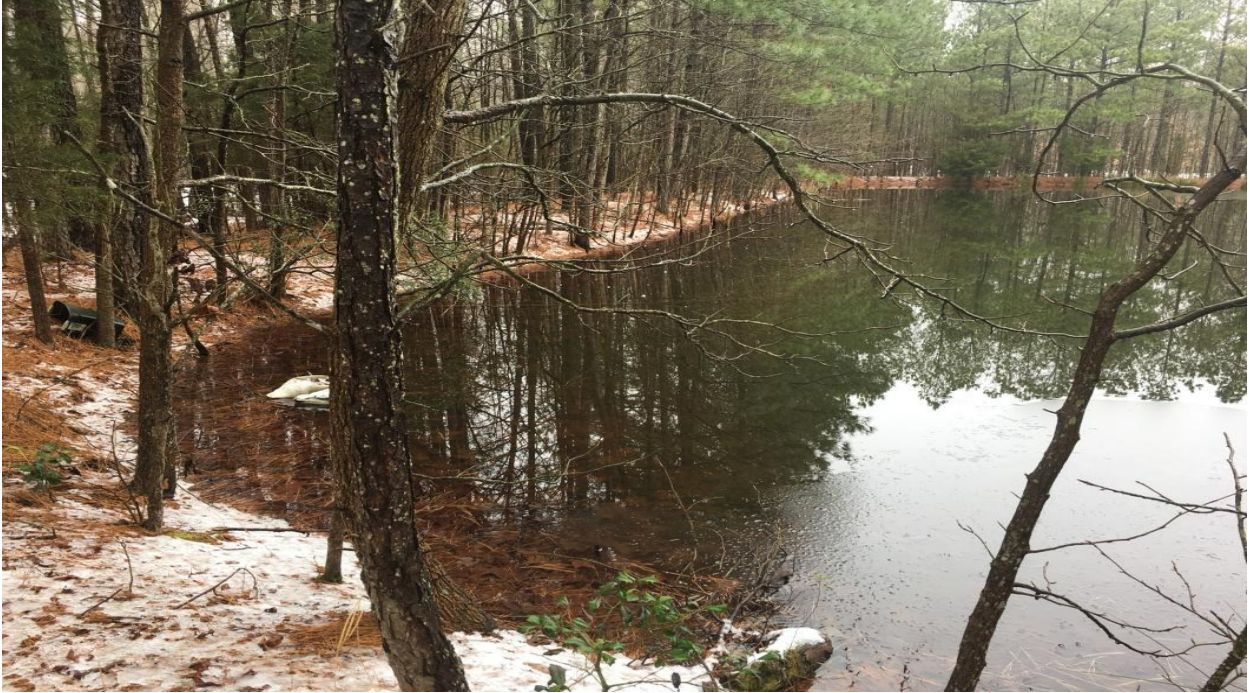
BIP with poor vegetation maintenance and less than 2 feet of freeboard.
