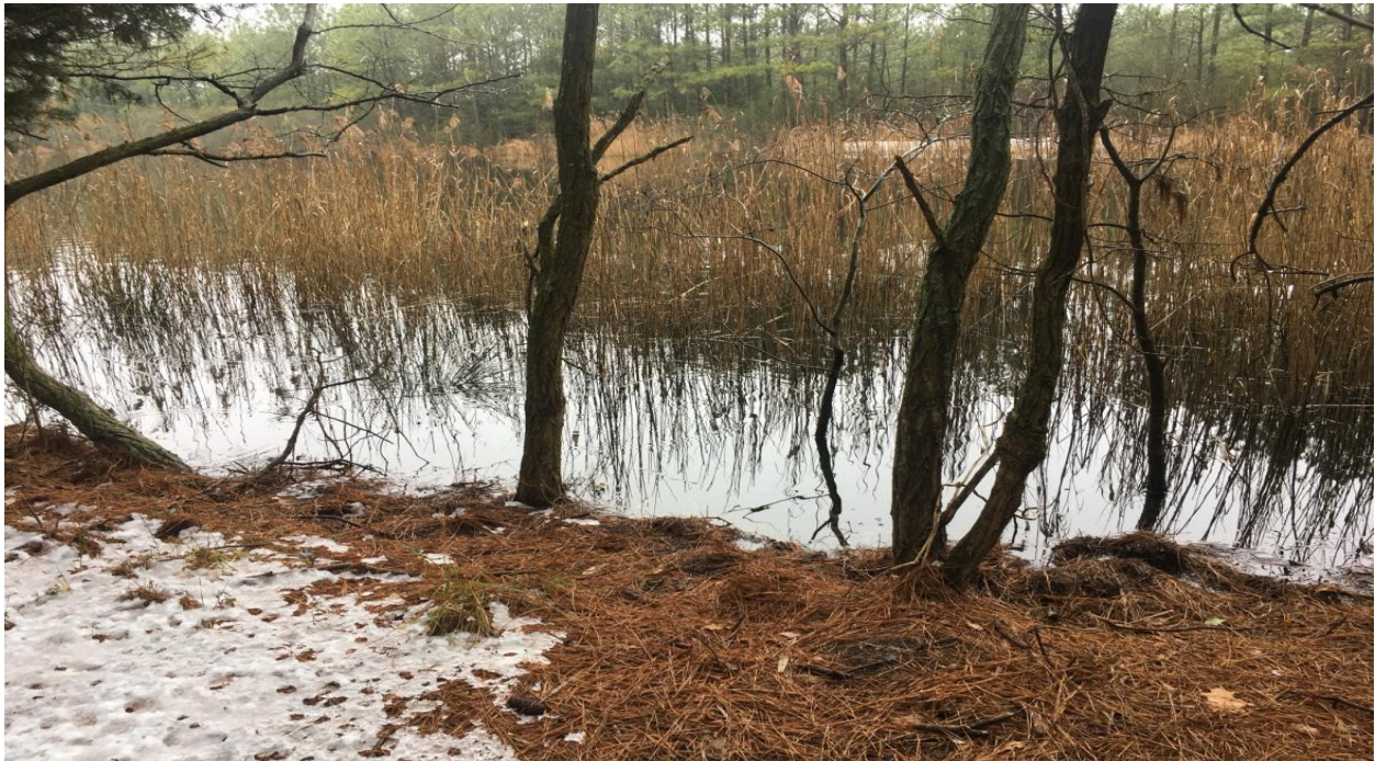
BIP with poor vegetation maintenance, lacking adequate fencing, and less than 2 feet of freeboard.
